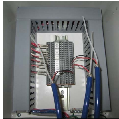
Figure 40: Level Transducer Connections
