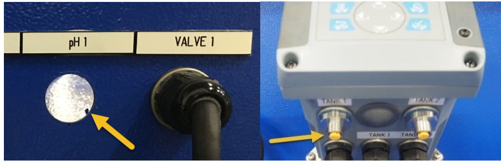
Figure 17 pH Probe Routing and Termination
